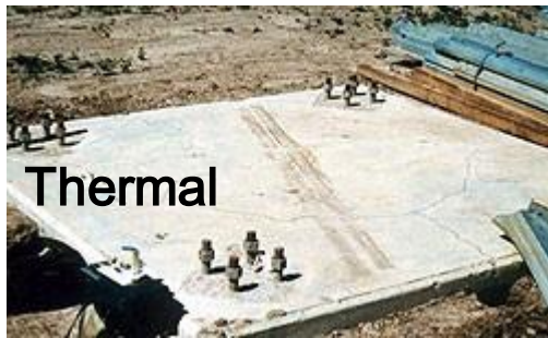
Freeze Thaw D Cracks
